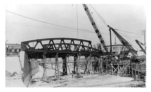
With Fairport's Main Street bridge temporarily closed for repairs, we look back 99 years, to March of 1914, and the construction of the lift bridge. The predecessor to the current bridge was an 80 foot long fixed bridge. In 1903 a decision was made to widen the canal to 125 feet, resulting in the replacement of bridges from the Hudson River to Lake Erie. Along the length of the canal, the widening occurred on the south side, leaving the towpath intact on the north shore.
