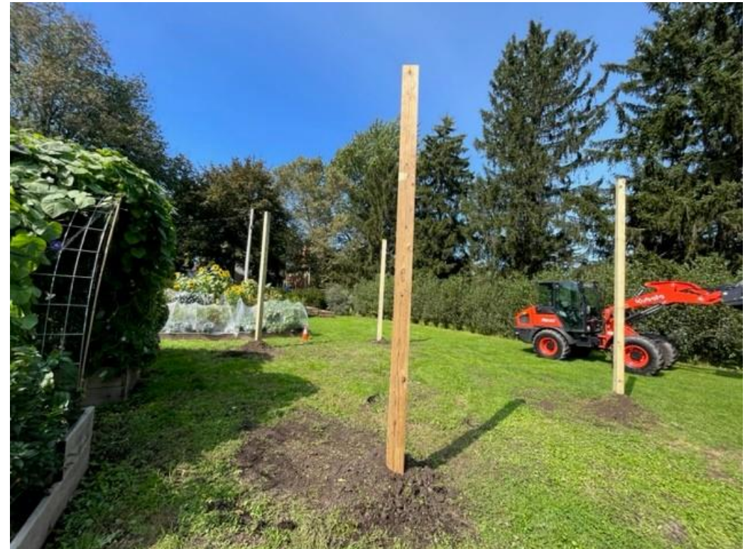
Install Posts for Shade Canopy
