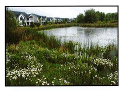
GOOD: This stormwater management pond with natural vegetation, reduces waterfowl and helps to clean stormwater.
