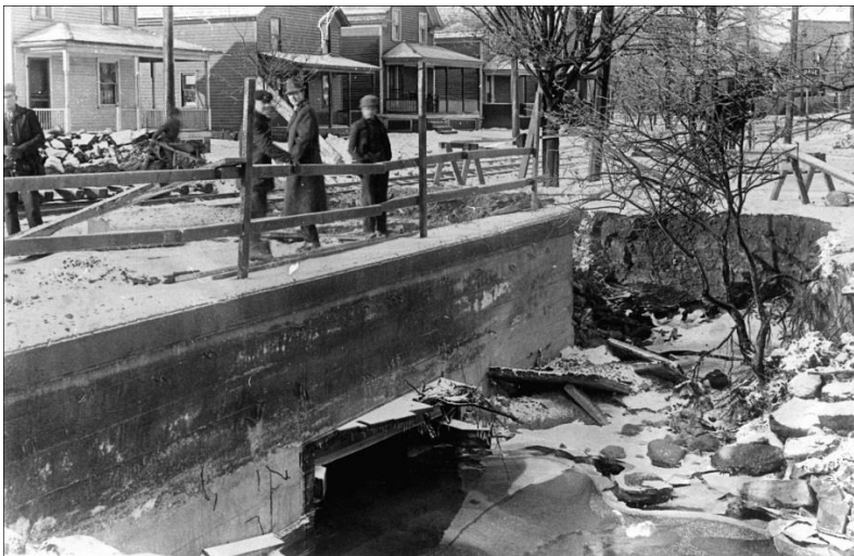
Men examine damage at the bridge at John Street caused by the flood of January 6 th , 1913. Rochester, Syracuse & Eastern trolley tracks can be seen running down John Street.
