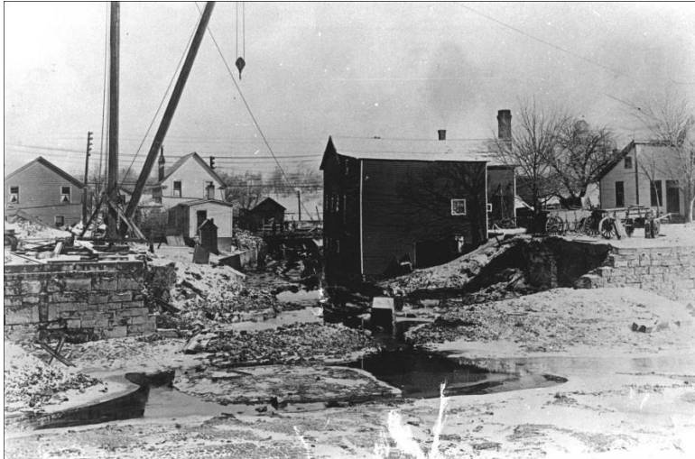
Image from January 9 th , 1913 of the washed out north wall of the canal at the waste weir, just west of the Parker Street bridge. The same location was the site of flooding in 2014.
